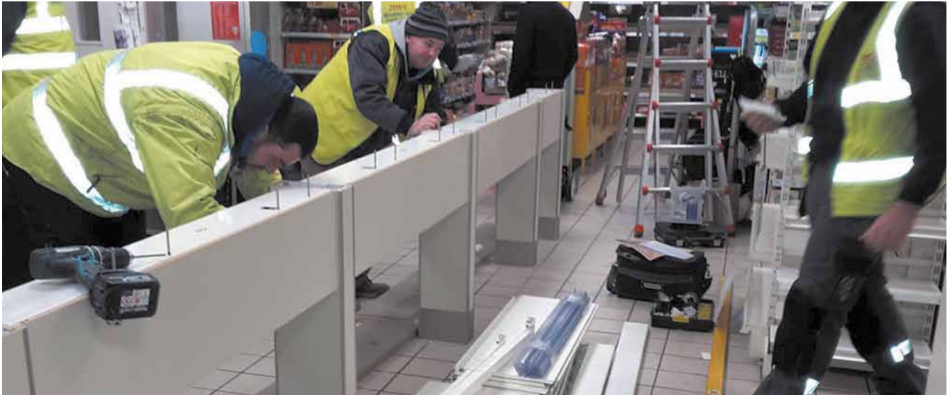
Installation by Displaymode in progress
